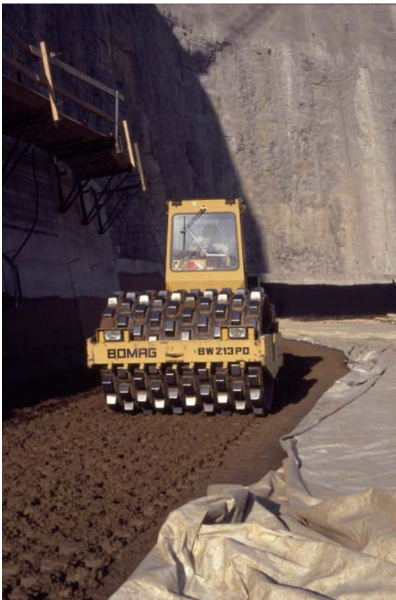
Photo 4: Kneading compaction by pad-foot roller
