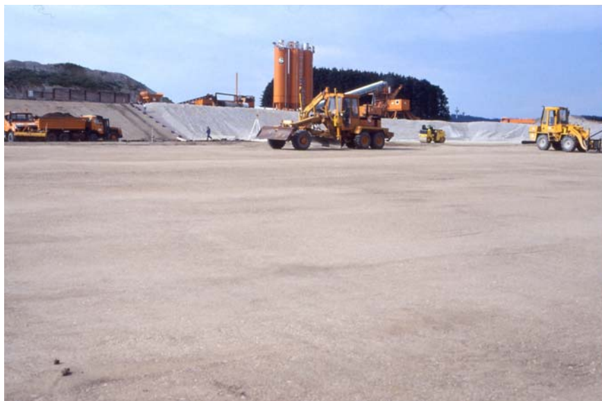
Photo 6: Mixed in-plant coarse grained well graded mineral liners
