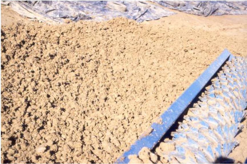
Photo 3: Homogenization of clay for compaction
